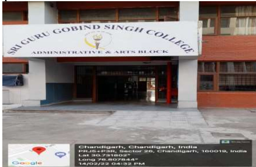
Ramp built for students and staff to access the main administrative block
